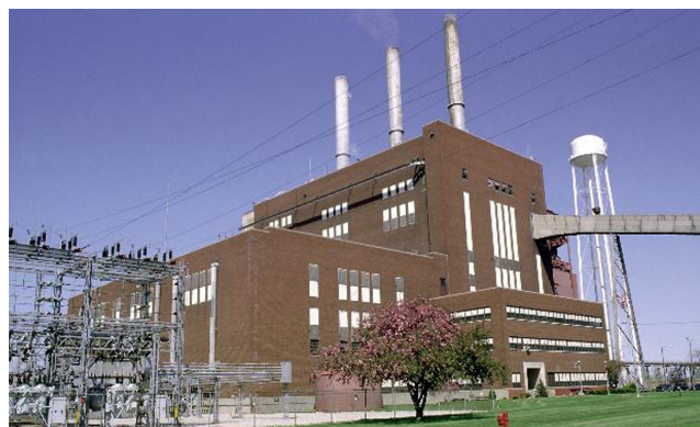
The J.R. Whiting Plant, one of Consumers Energy's "Classic Seven" coal plants slated for retirement. (Source: Consumers Energy)
